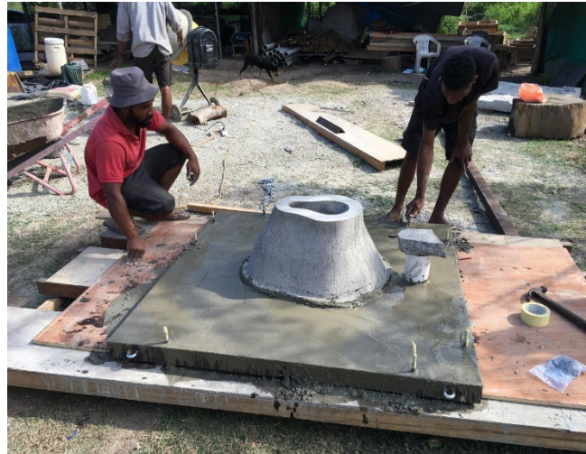
Figure 4 - Sliding Latrine slab being cast
